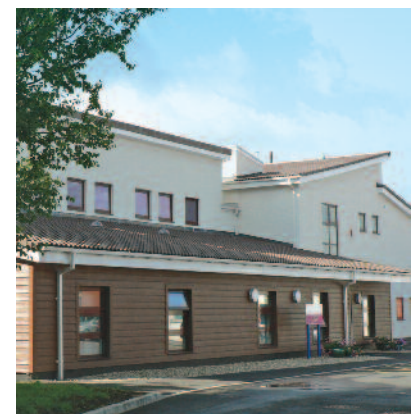
The BCRM building at Southmead Hospital
